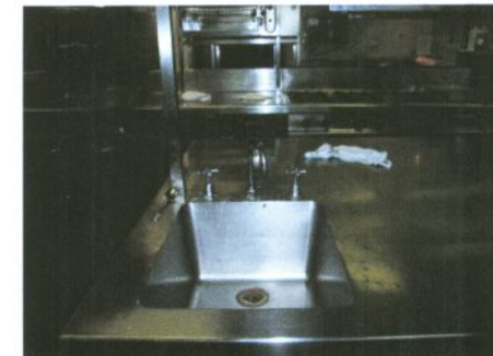
Installed kitchen Tap Restrictors
