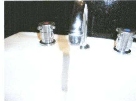
Install Basin Tap Restrictors on Bathrooms
