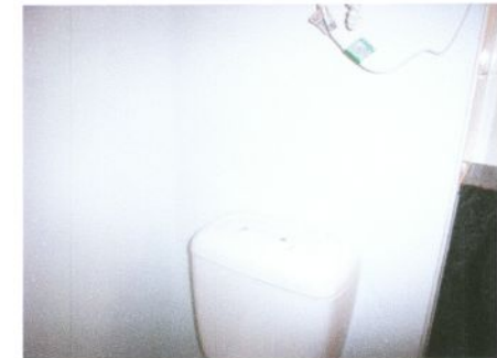
Installed Dual Flush Cisterns
