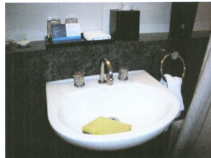
Installed Guest Room Tap Restrictors
