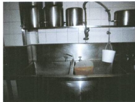
Install Basin Tap Restrictors in Kitchen
