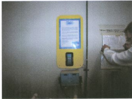
Installed 'Anti-Bio' System to Pool
